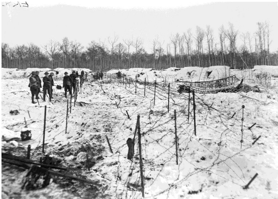
Image 1: A party of the 22nd Battalion constructs apron wire entanglements, Ploegsteert Wood, Belgium, 26 December 1917.
