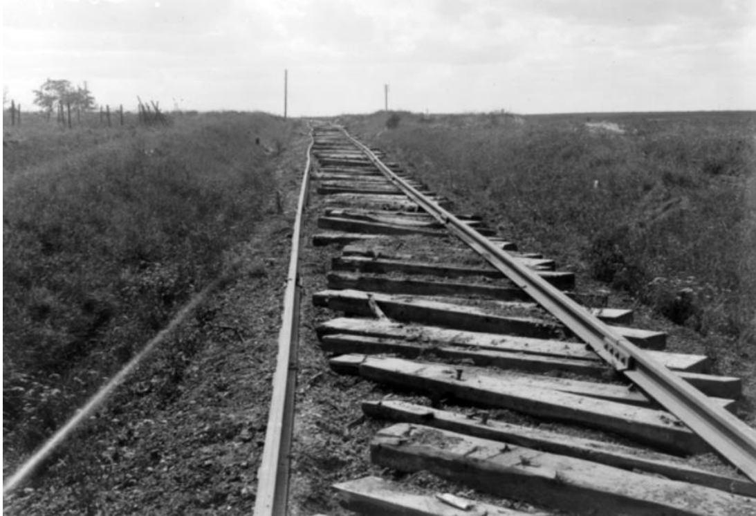
Figure 1: View of the railway near Halle, illustrating the German method of shifting sleepers to sabotage the line (AWM E03241)
