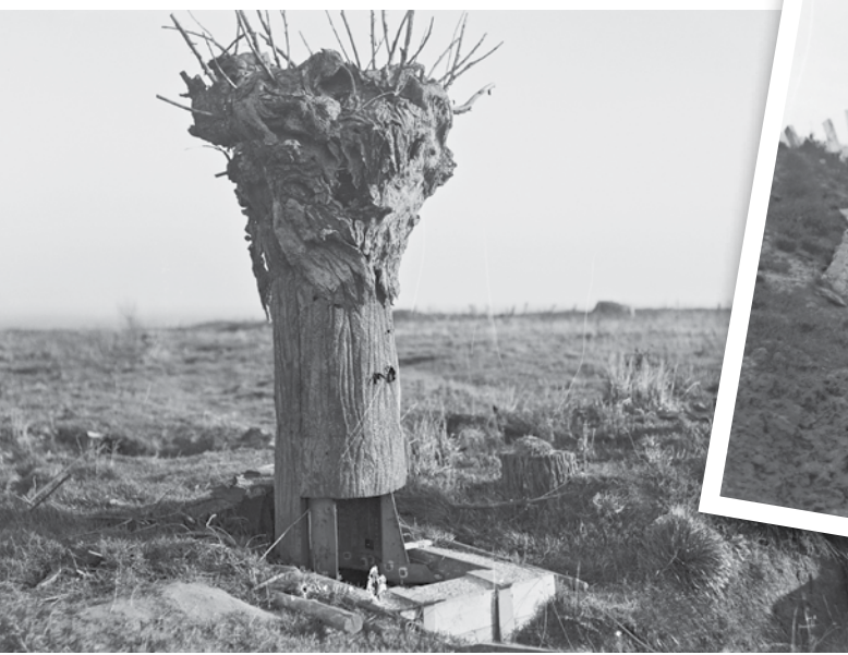
“Dummy” trees were used as observation posts on the battlefield. This one was built in the Messines area in December 1917.
