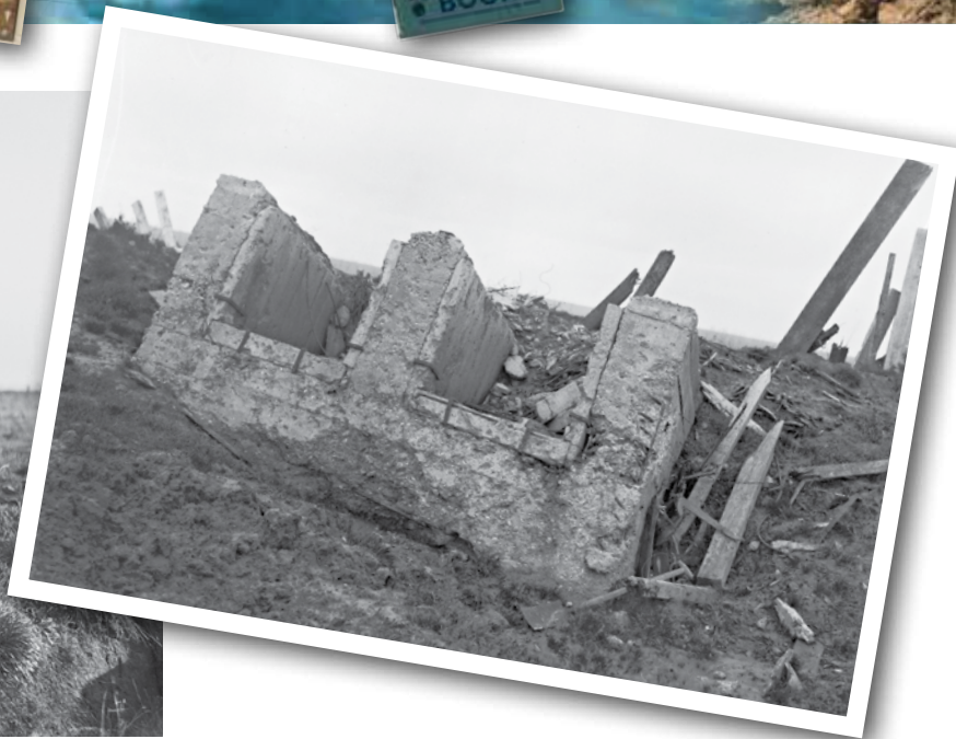
This concrete pillbox was overturned by the force of the underground explosion at Messines in Belgium.
